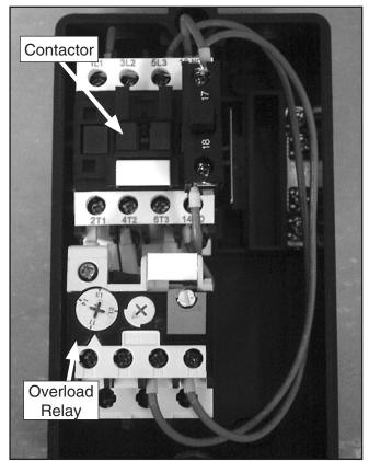
Figure 88. G0588 3-phase magnetic switch.
